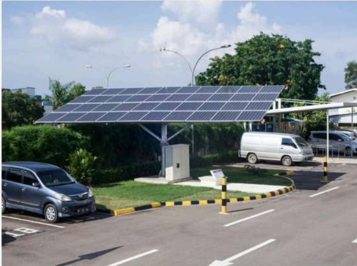
Solar Tracker System-Panasonic Batam
